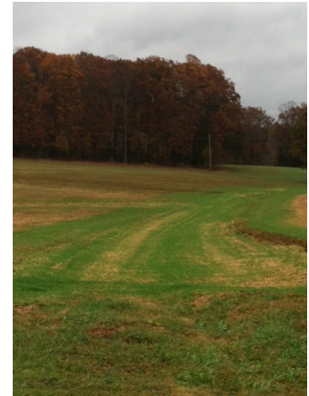
Newly completed Grassed Waterway
