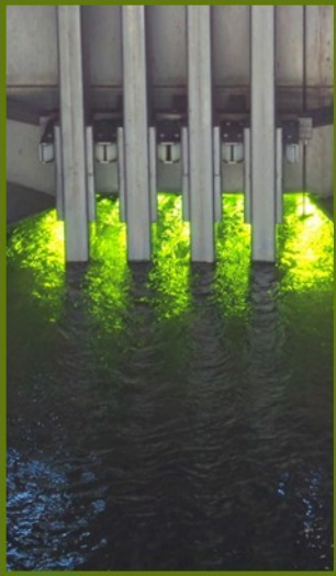
Ultraviolet (UV) System
