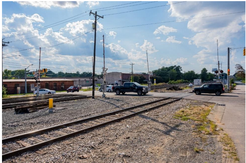
Figure 7: Driver Street Crossing
