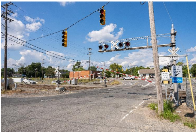
Figure 23: Ellis Road Crossing – Looking North
