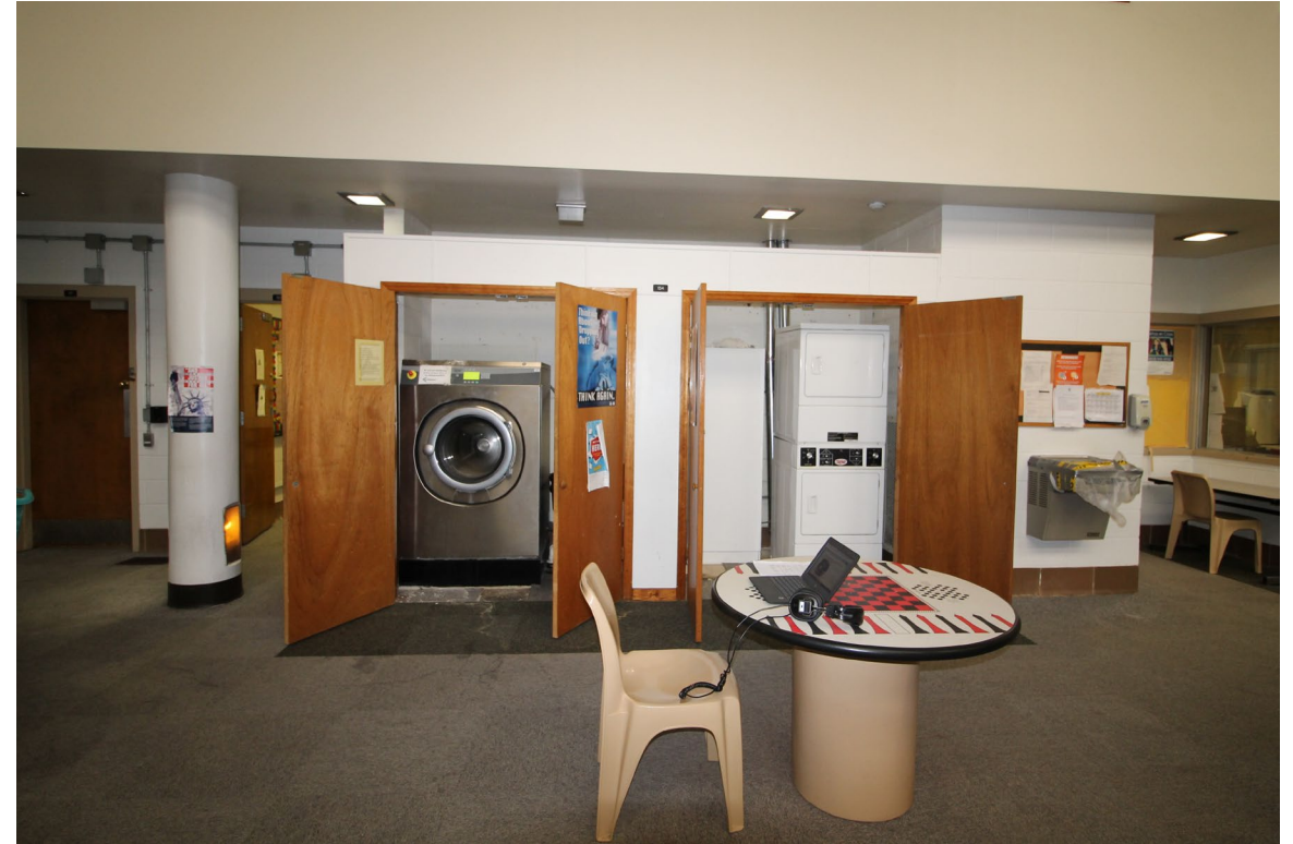
LAUNDRY FACILITIES (INSIDE DAYROOM)
