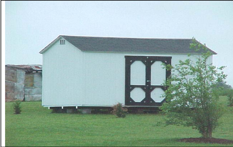
MS 17 STORAGE BUILDING
