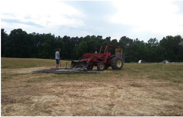
Automatic Waterers- construction
