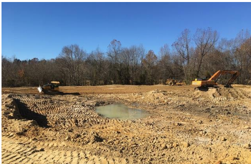
AgWRAP- pond construction
