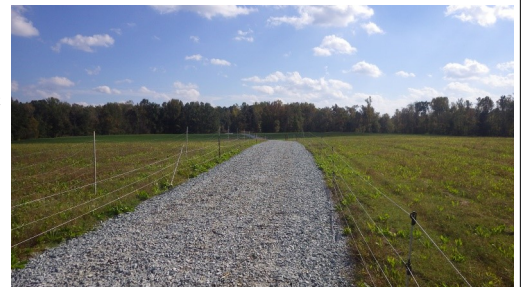
Animal Trail and Walkway under construction
