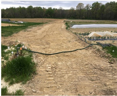
Grassed waterway mid construction
