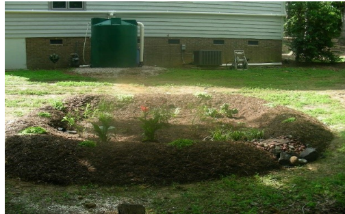
Pictured above: Rain garden and cistern
