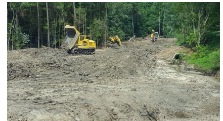
Construction on Southern High Project/Phase I- Summer 2016
