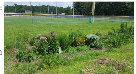
Southern High- bio-retention basin
