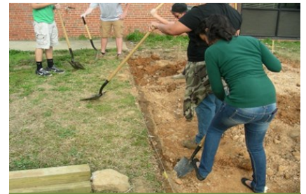
Students and volunteers at work on the wheelchair accessible garden at Northern
