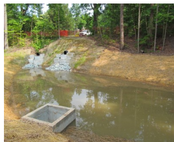
After Forebays installed to decrease velocity storm events
