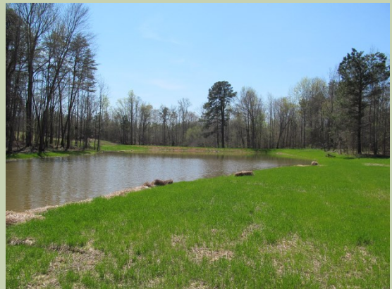
After Pond Installation
