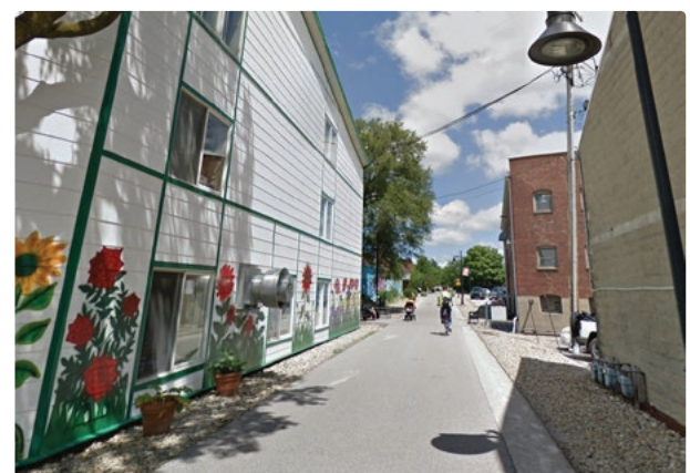
After the opening of the B-Line Trail, an existing business (left) added a walk-up window oriented toward the trail. On the right, new mixed-use development oriented to the trail. Bloomington, IN.
