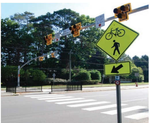
Example of trail crossing with user-activated stop light (Pedestrian Hybrid Beacon)
