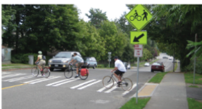
Pavement markings & signs
