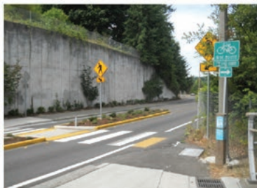
Raised median island Restrictions: where space allows
