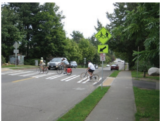
Example of trail crossing with pavement markings and signs
