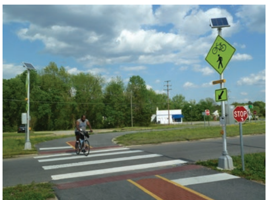
Example of trail crossing with User-activated flashing sign (Rectangular Rapid Flashing Beacon)
