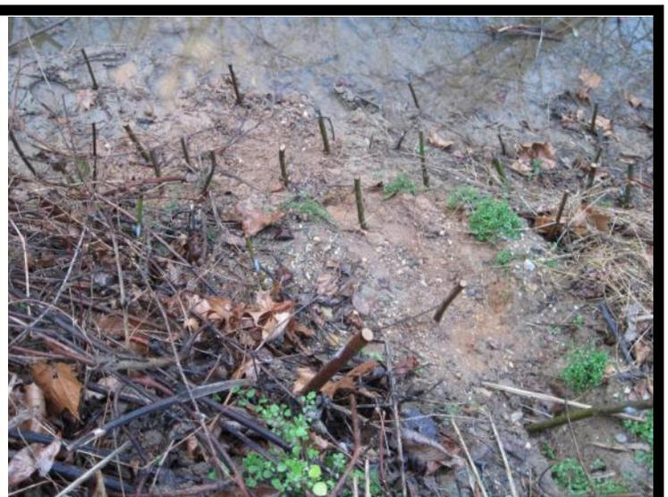
*Option 2: Plant diverse, native flora without changing the grade (above left illustration). Above right photo shows livestakes installed every 1' on existing slope to create snag and quick root mass (© N. Alexander).*
