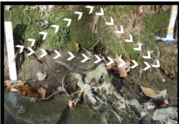
**Step 3:** Plant first row every 3' minimum. Stagger another row a few feet up in a triangular pattern and begin again. As long as the soil is saturated, livestakes can be installed.
