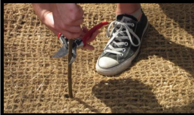
**Step 2:** Orient livestake with leaf buds facing upward (pointed end goes into the ground). Hand push or gently hammer livestake  $\frac{3}{4}$  of the length into the bank. Make sure to leave 3"-4" sticking out of ground above soil line. If the top of the stake is smashed, make a clean cut for faster and healthier healing of the livestake.
