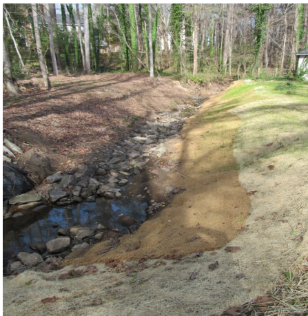
After streambank stabilization.
