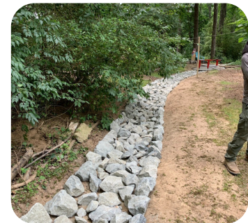
Structural Stormwater Conveyance
