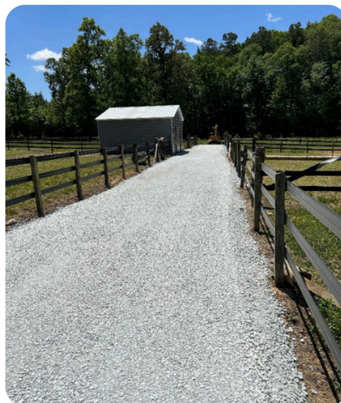
Ag Road Repair
