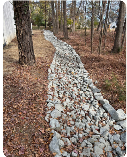
Stormwater Conveyance Latta Rd Project
