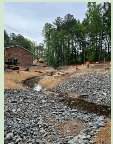
Project In Progress
