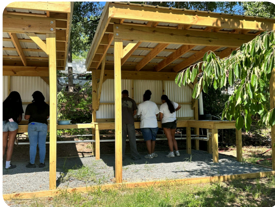
Left: Wash Station
