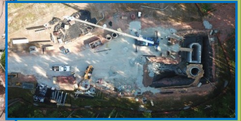
Shiloh Glenn Progress
