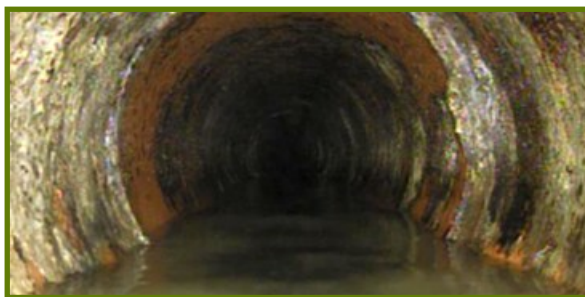
CCTV view of grease lined sewer pipe
