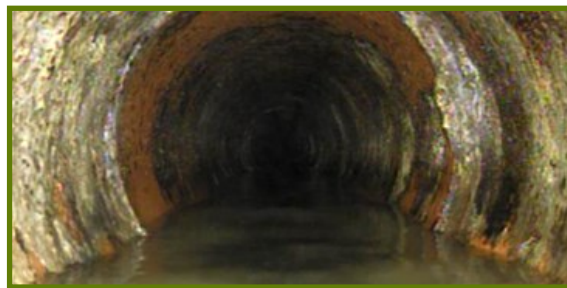
CCTV view of grease lined sewer pipe
